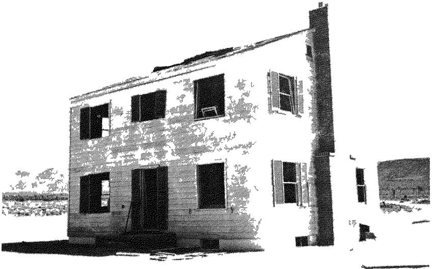
Figure 4.16 Wood-frame house after the nuclear explosion (1.7 psi over pressure)
